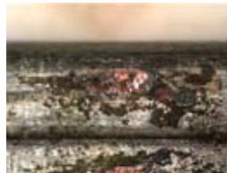
Micromotion causes fretting of the male and female contact surfaces. This eventually leads to corrosion that can interrupt current flow. Contact lubricants cushion the motion and protect the contact from fretting.
